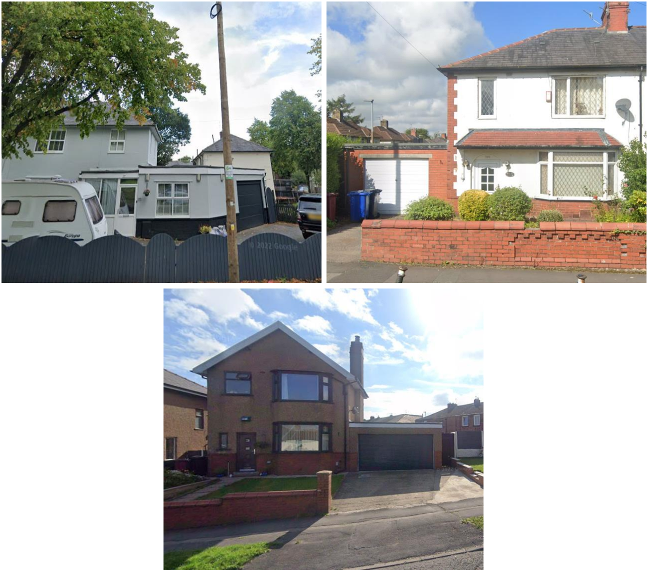
Figure 4: Existing Flat Roof Side Extensions (Left Top – 77 Green Lane, Right Top – 106 Shorrock Lane, Middle Bottom – 221 Shorrock Lane)
